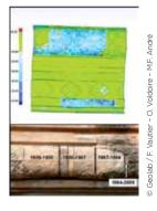
3D mapping of the damaged areas and photographs taken at different dates: large erosion scars have formed since the temple was cleared of its forest canopy, erasing all traces of the ornamented surface
