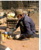
Preparing structural adhesive for stone repair
