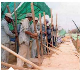
Compacting the soil on the western causeway, 2005
