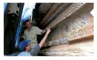
Eastern façade of Ta Keo: the use of short-range laser scans allows for 3D modelling of sandstone decay
