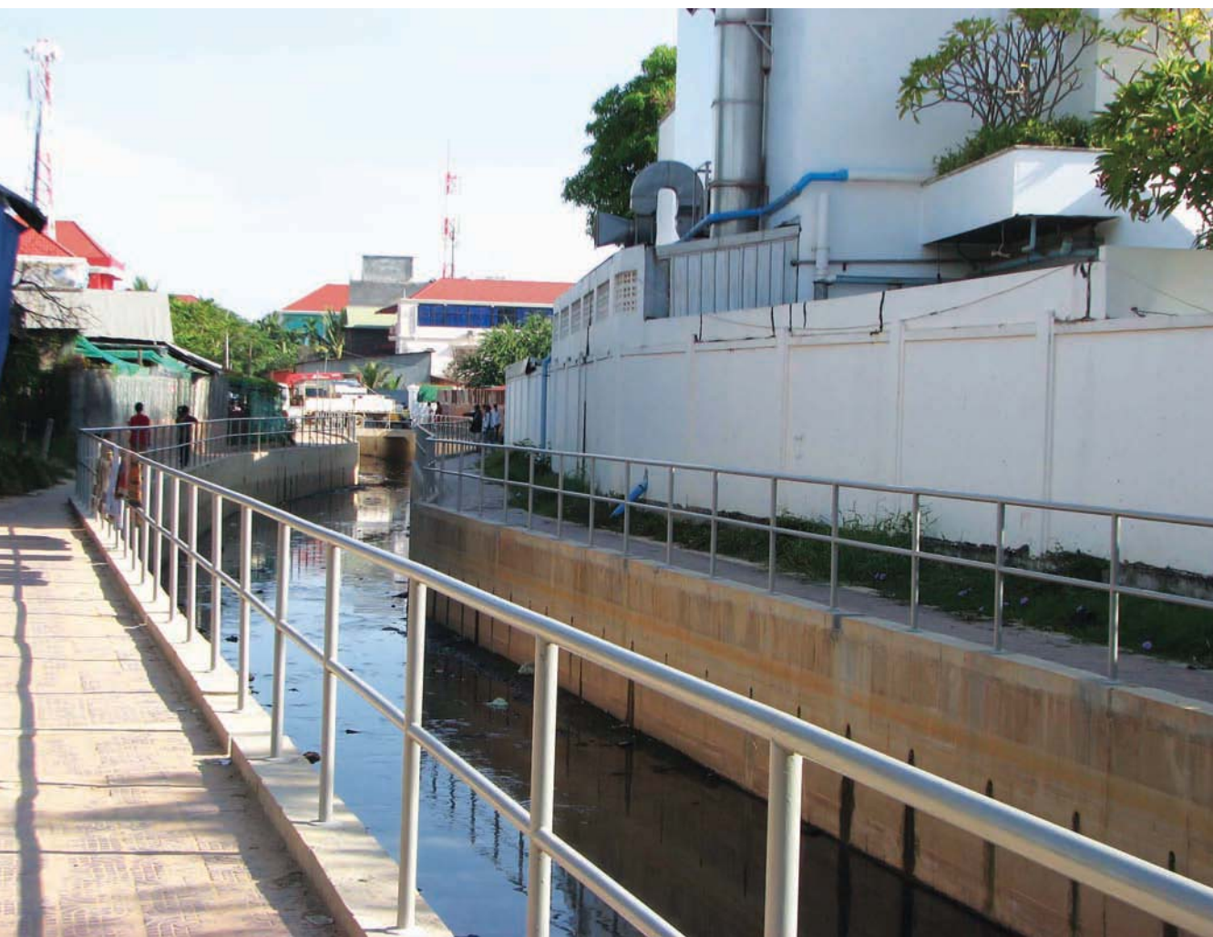
Waste water disposal line - Siem Reap town
